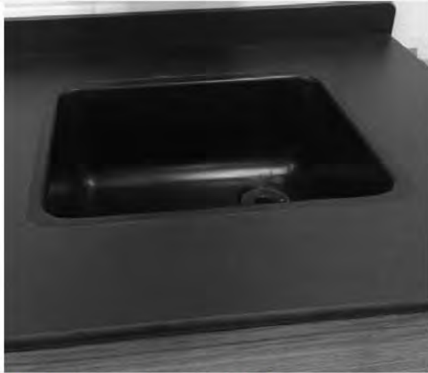
HPL Surface, Backsplash, and Sink
