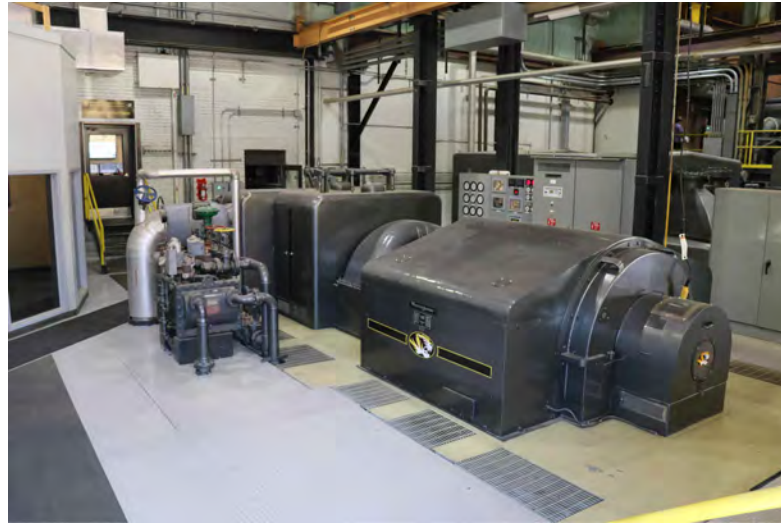
EXISTING TURBINE 6 (LOOKING NORTH WEST)
