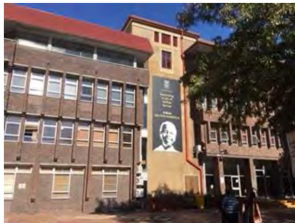
University of Western Cape Administration Building.
